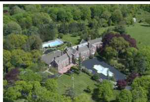
Dunnellen Hall Greenwich, CT $75,000,000
